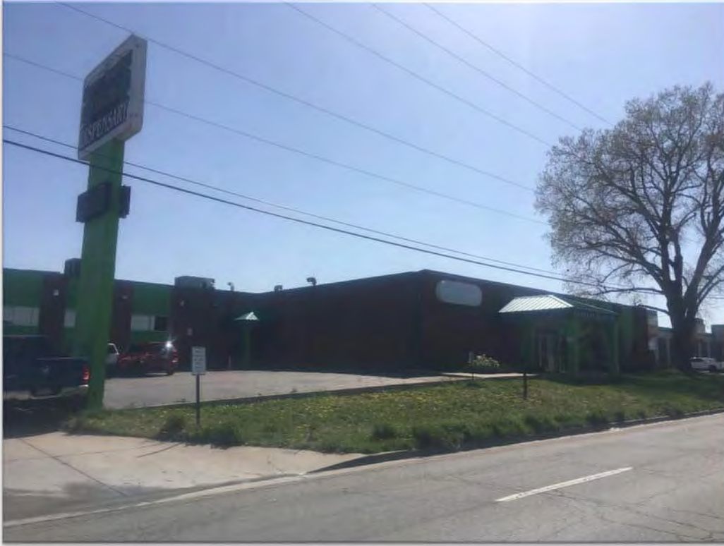
5DV34927_3: North (primary) elevation and west elevation. The dispensary sign is shown at left.
