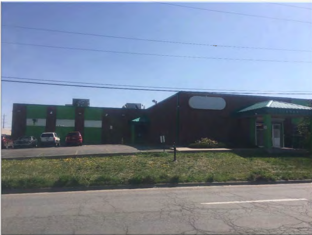
5DV34927_4: North (primary) elevation and west elevation.
