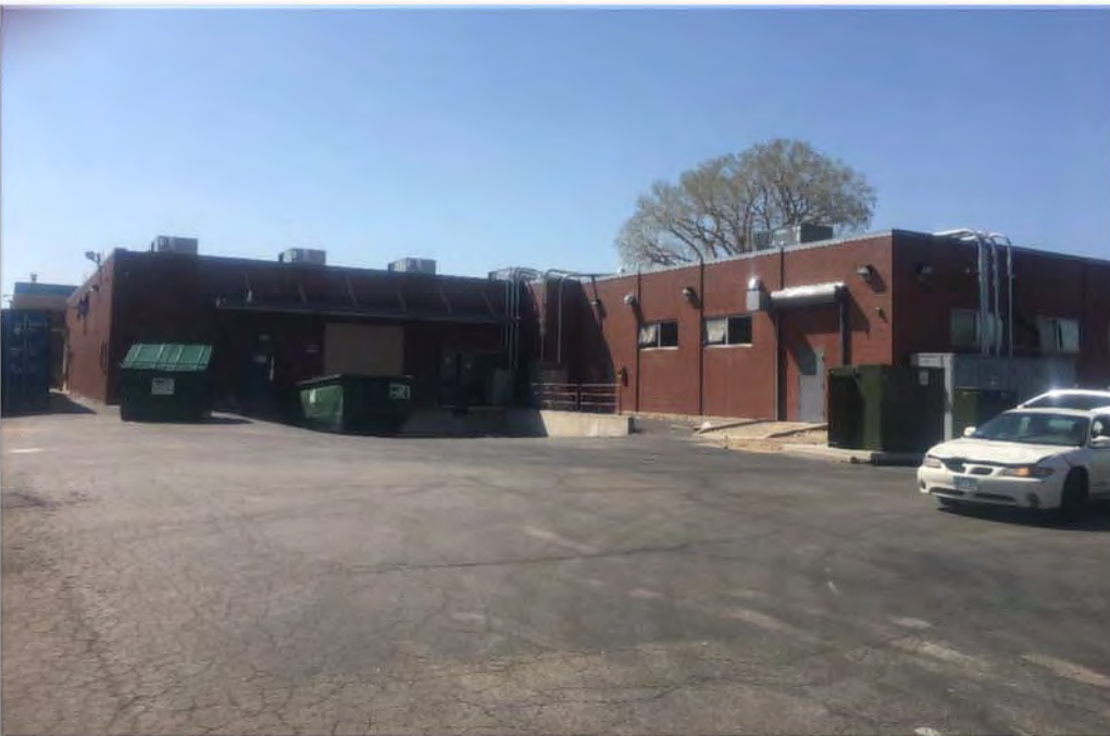
5DV34927_6: South (rear) elevation.
