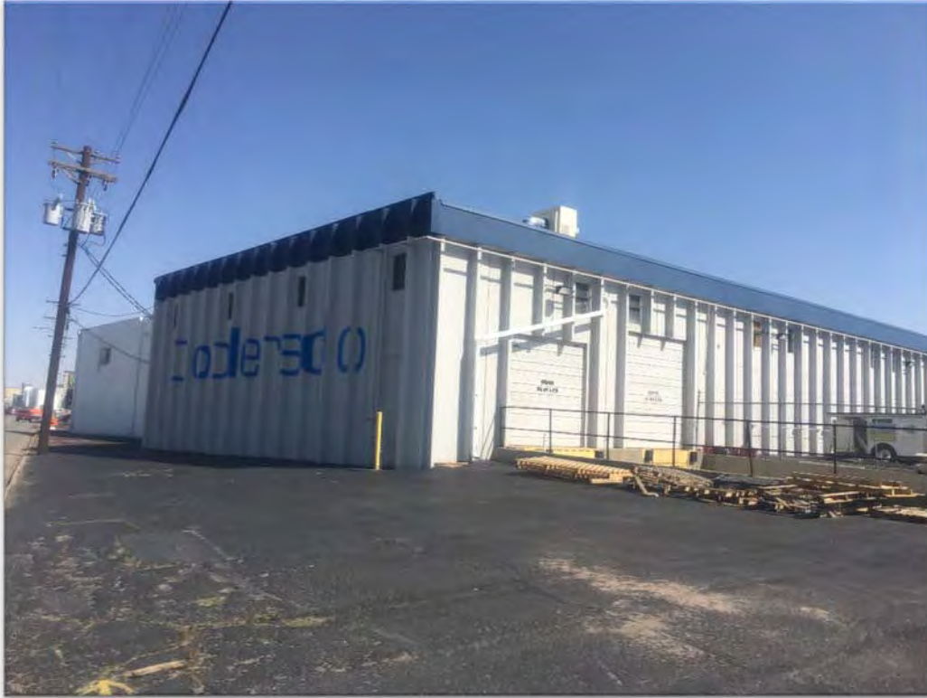
5DV34925_1: North and west elevations. The "Coolerado" name is on the north elevation.
