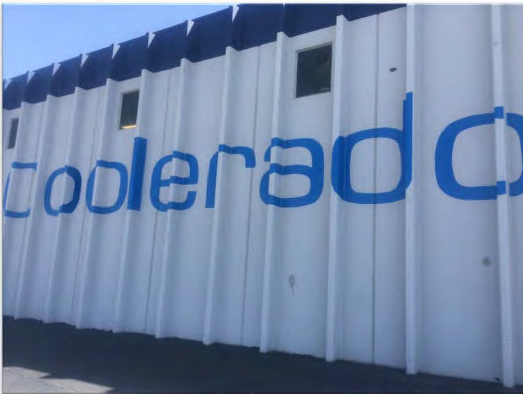
5DV34925_6: Detail view of the "Coolerado" name on the north elevation.
