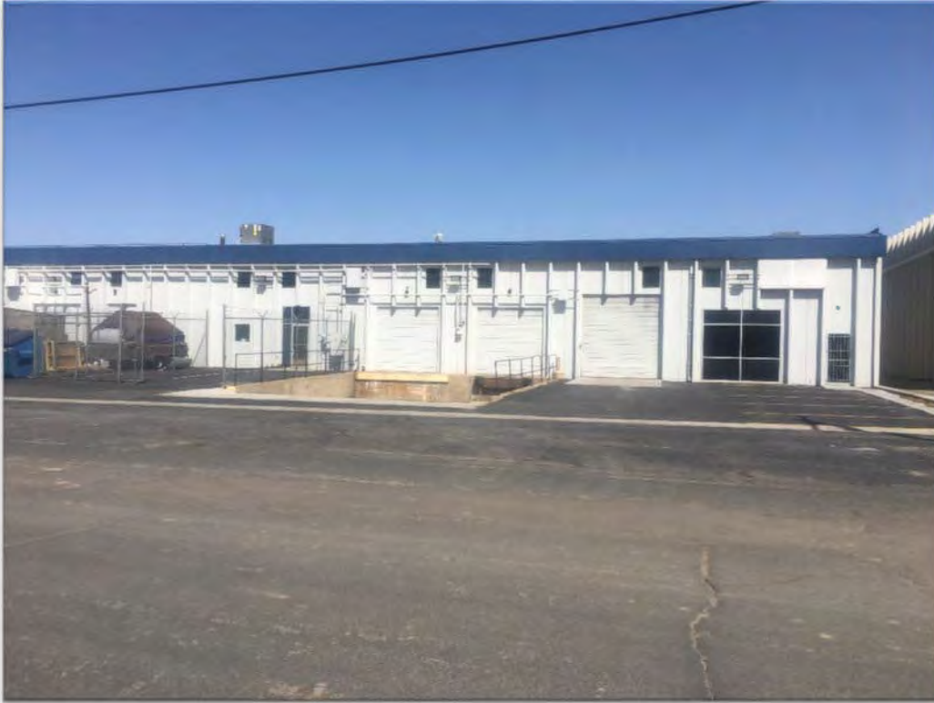
5DV34925_3: South end of the west elevation. View: East
