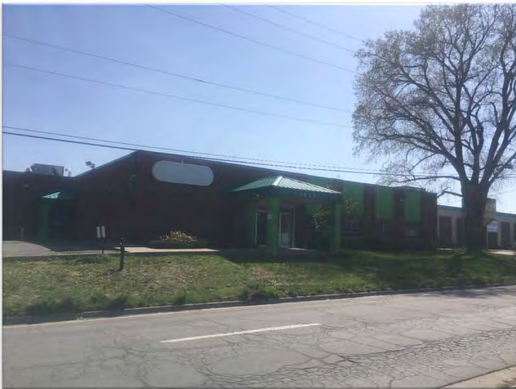
5DV34927_2: North (primary) elevation and part of the west elevation.
